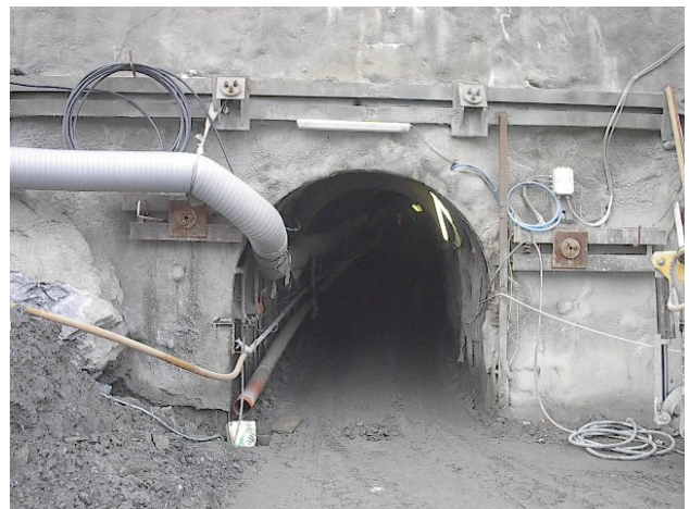
Figure 4 – The tunnel entrance during construction
