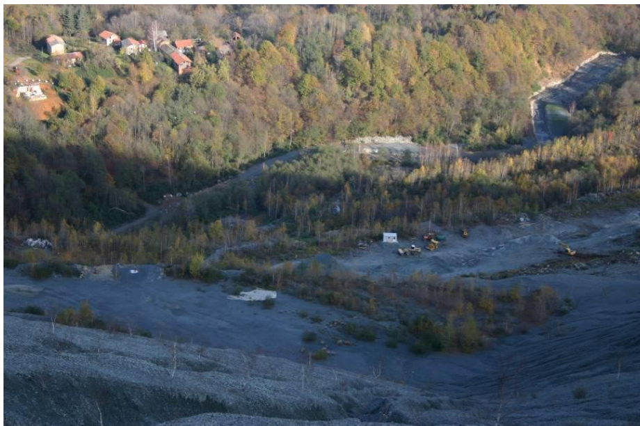
Fig. 2: Looking down slope: nearby houses, the Fandaglia Creek and the decant basin
