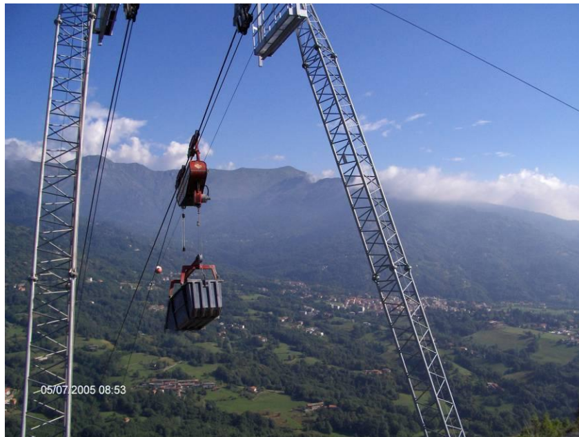
Fig. 4: Aerial Tramway for hauling down material. Braking of the tramway produces electricity which is sold to the grid.
